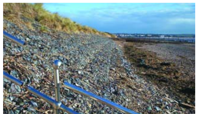
Image 7k: Rock gabion exposure after the storm of October 2004 Source: Exe Estuary Management Partnership
