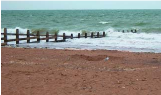
Image 7c: Wooden groyne at Dawlish Warren Source: Exe Estuary Management Partnership
