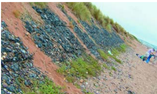
Image 7j: Rock gabion exposure prior to south easterly gales Source: Exe Estuary Management Partnership
