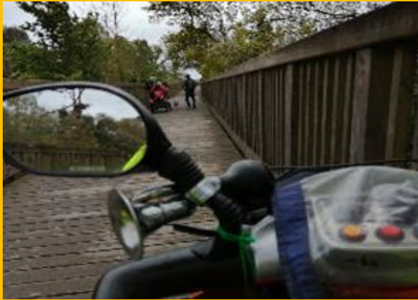
Photo 1. Exe Estuary Trail wooden boardwalk
